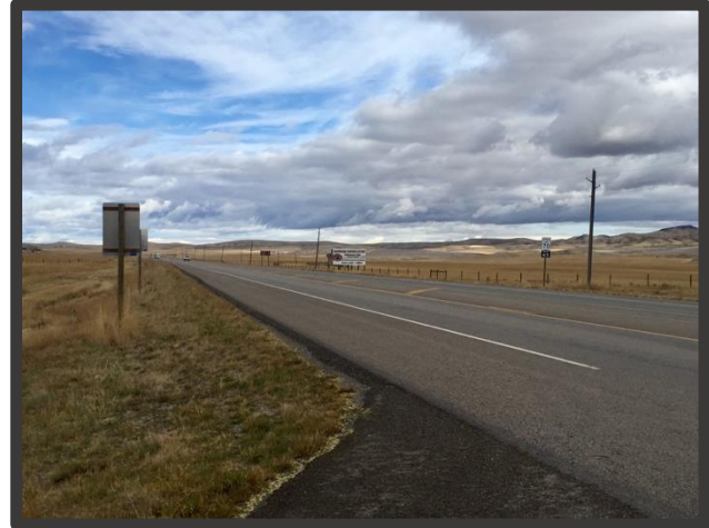
Figure 6. Highway 287, north of the I-90 Interchange
