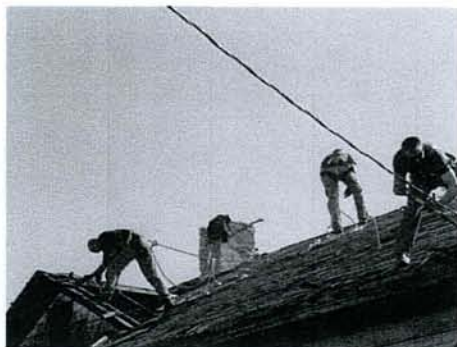
Remove & repair roof
