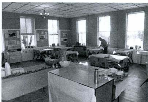
Install suspended ceiling in Community Room (South Room)
