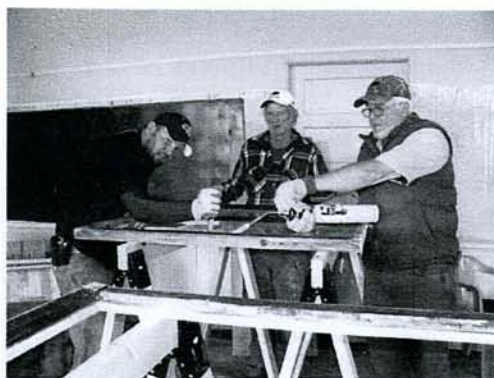
Window Repair/Glass Replacement
