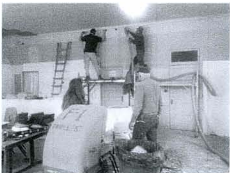
Insulate walls/ceiling
