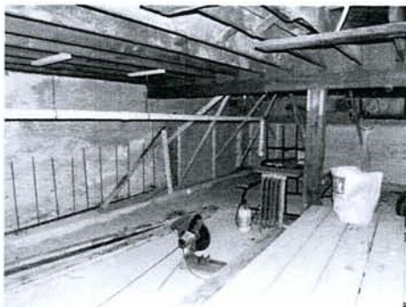
Upgrade basement foundation/walls
