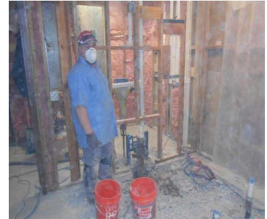
Corroded water pipes under concrete floor
